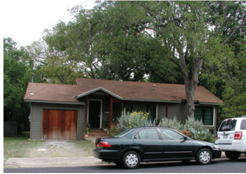
A SQUAT, ONE-STORY, NONDESCRIPT HOUSE (LEFT) IN THE ROSEDALE NEIGHBORHOOD OF AUSTIN, TEXAS WAS REINVENTED INTO THE SILVER AGAVE HOUSE (RIGHT), A MODERN, TWO-STORY BEAUTY.
